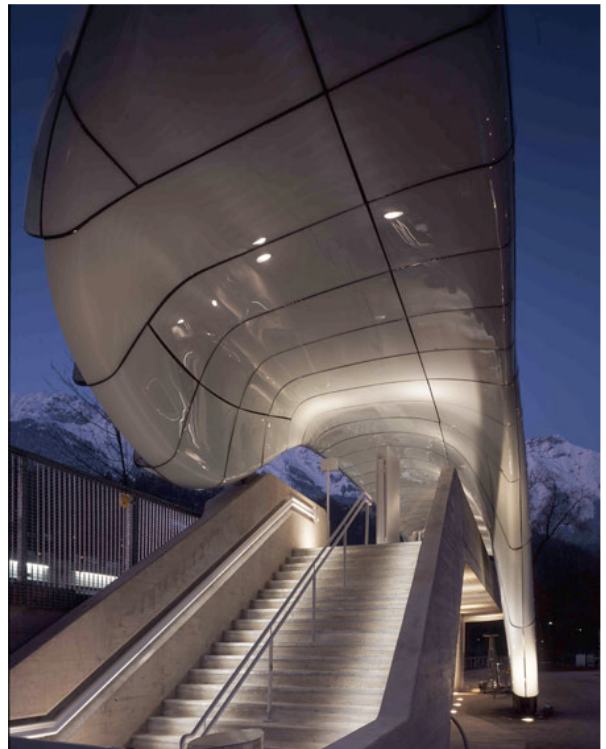
Above: Zaha Hadid's new signature designs at the Nordpark Cable Railway Stations in Austria set the global benchmark for the use of double curvature glass in construction. Continued on page 5.
